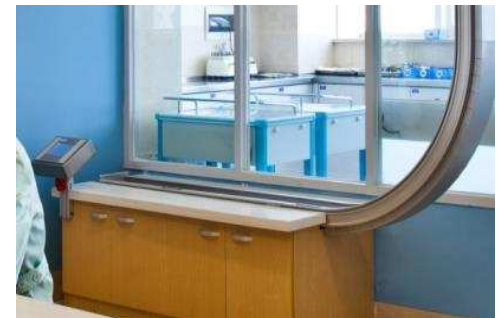
Re-entry station for average capacity 40 transports/ hour
